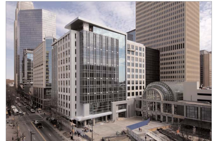
Exterior work almost complete at The Main.
