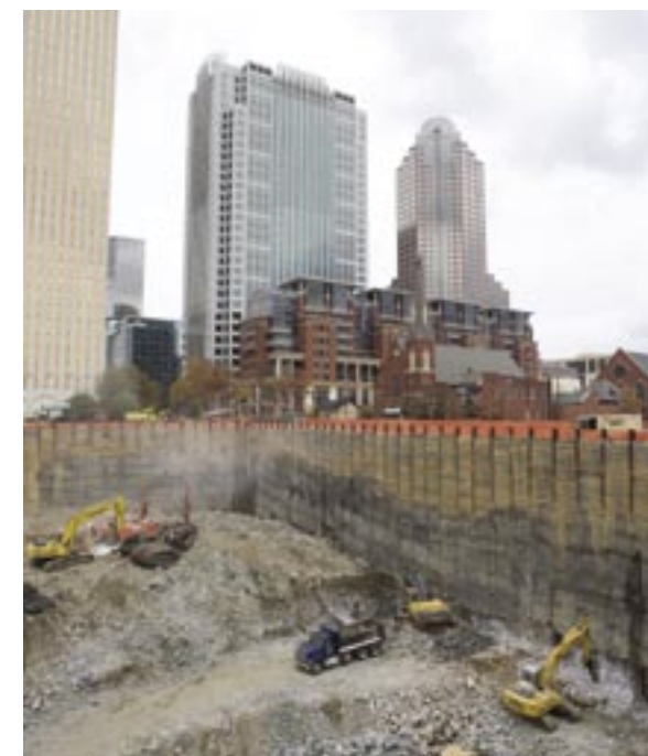
Trucks will haul away 400,000 cubic yards of materials after the blasts.
